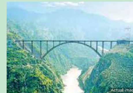
Chenab Railway Bridge, Jammu & Kashmir 2023
