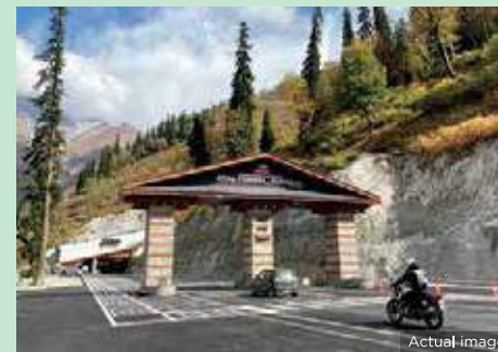
Atal Tunnel, Himachal Pradesh 2020
